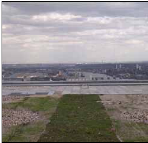
Figure 2 Barclays Tower, Canary Wharf
