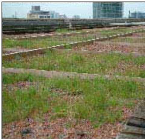
Figure 4 Canary Wharf Green Roof Laboratory
